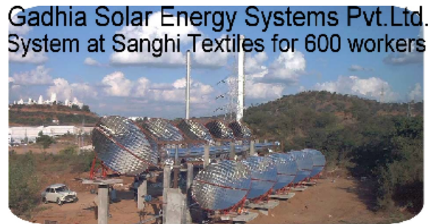
Picture 3: System at Sanghi Textiles for 600 workers
